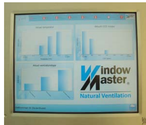
Fig. 3.63 Computer monitoring and regulating system for regulating the building's energy consumption
