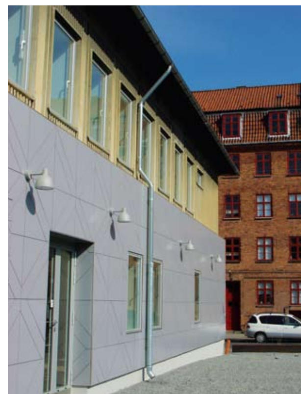
Figs. 3.64a & b Extra insulation of facades
