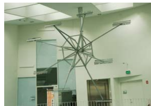
Fig. 3.58 Art piece on the top floor for reflecting the sunlight from the roof
