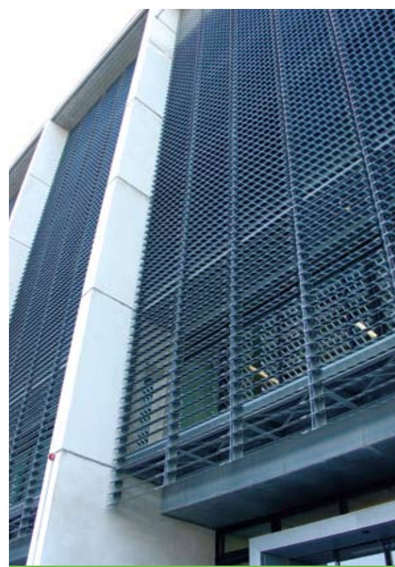
Fig. 3.71 Adjustable solar panels on headquarters of Copenhagen Energy
