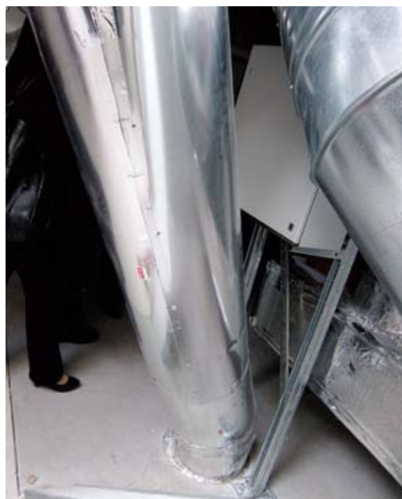
Figs. 3.60a & b Aluminum pipe with reflective glass inside
