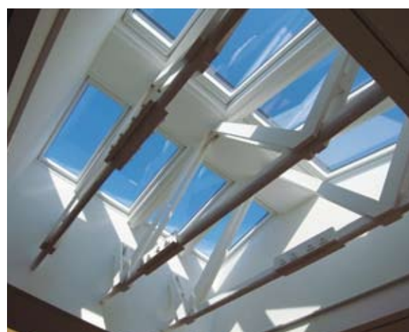
Fig. 3.62 Daylight utilization through window installed on the roof
